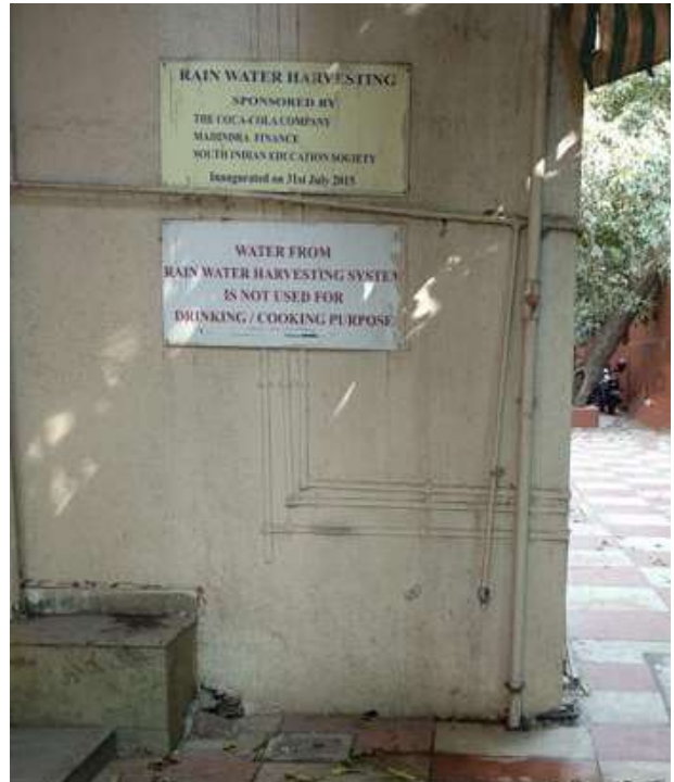
Rain Water Harvesting
